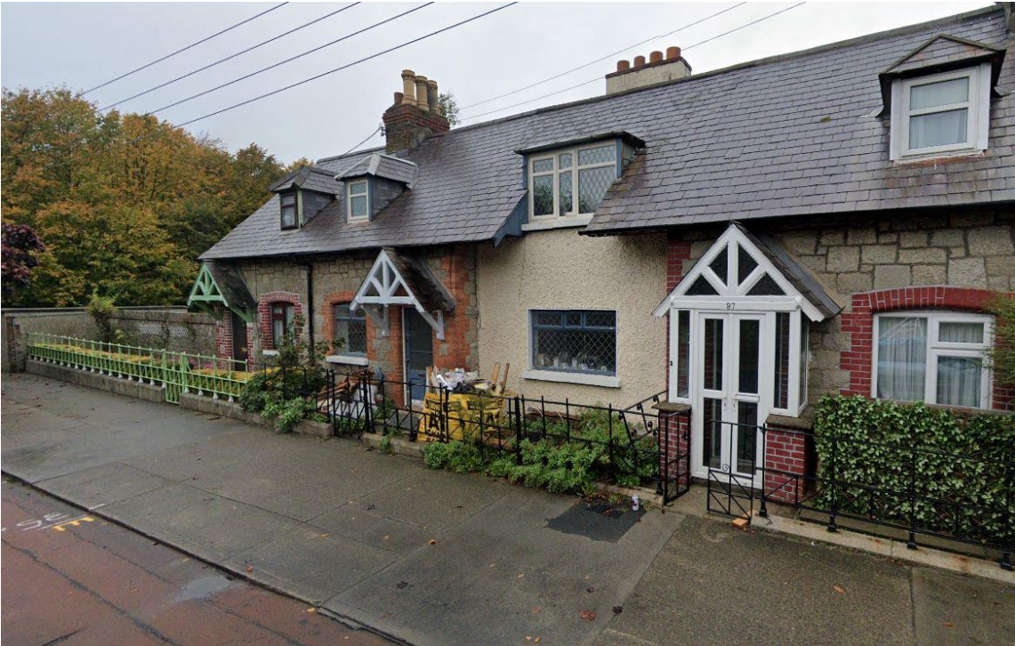
Figure 15: Photograph of Castle Cottages, Roebuck Road
