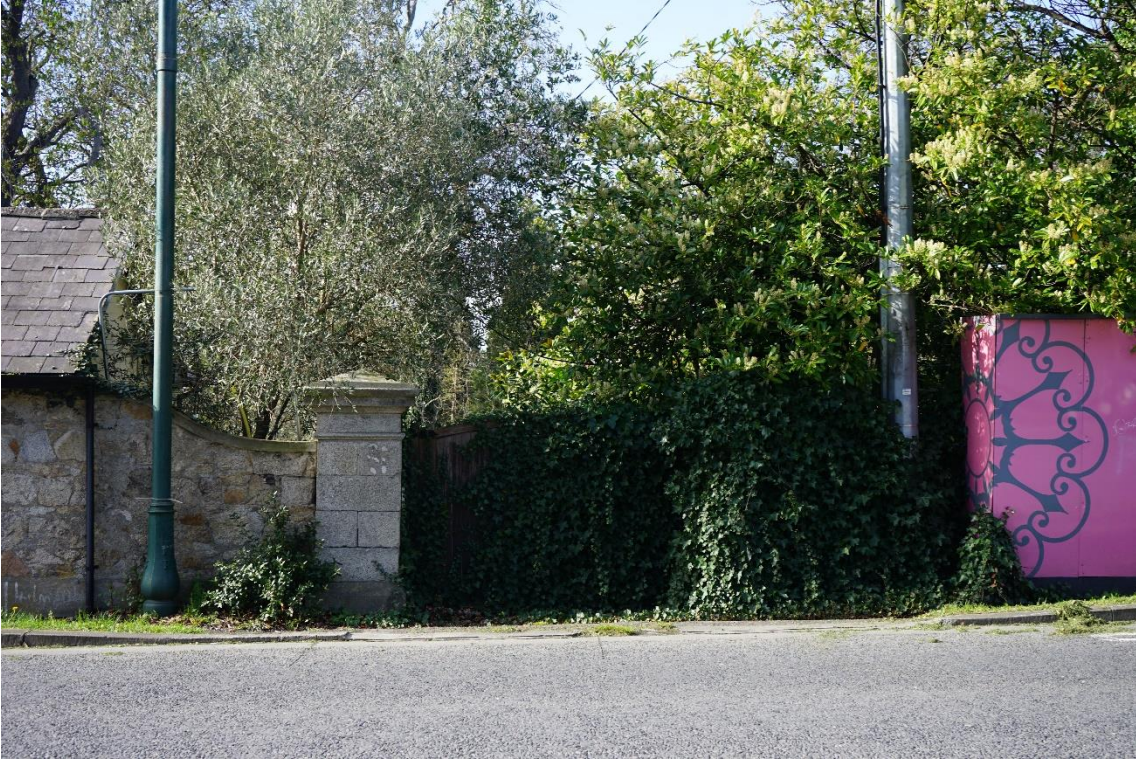
Figure 3: Lodge entrance, Protected Structure No.740
