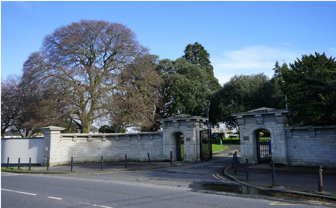
Figure 6: Photo of entrance into Sacred Heart Convent, Mount Anville
